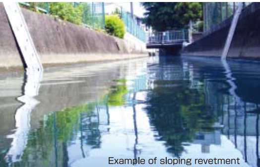
Example of sloping revetment
