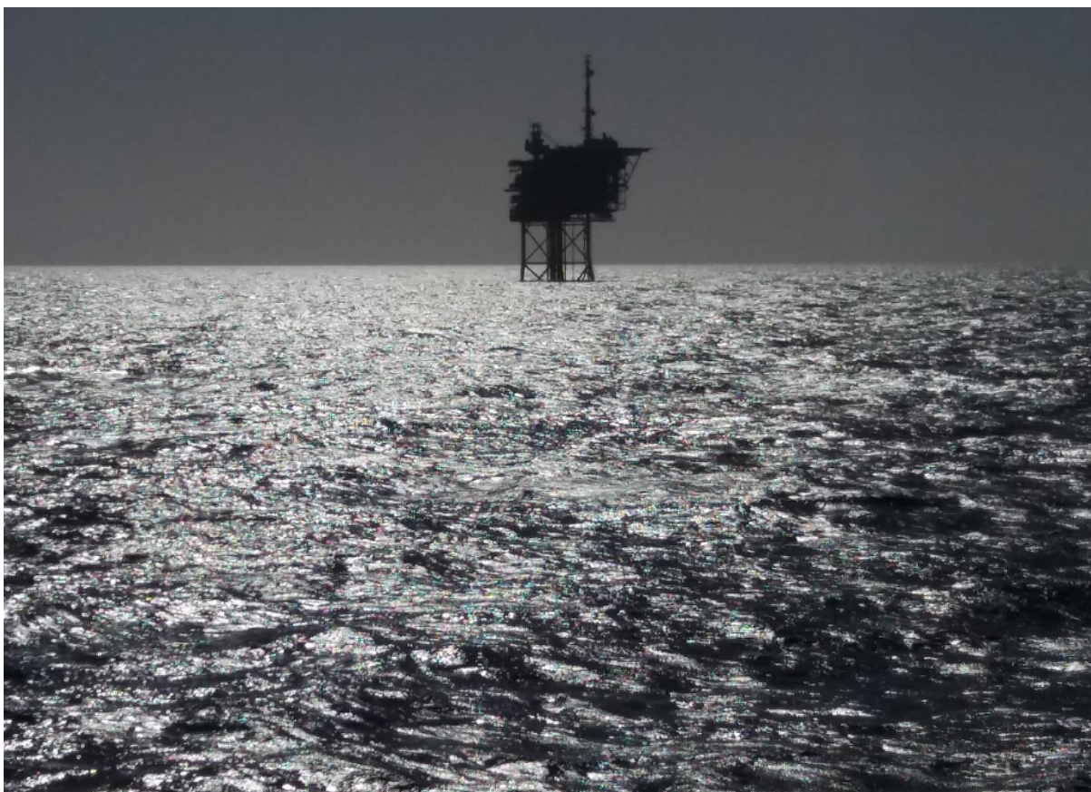
Figure 4.9: Platform A12-A. Photo Henko de Stigter.
